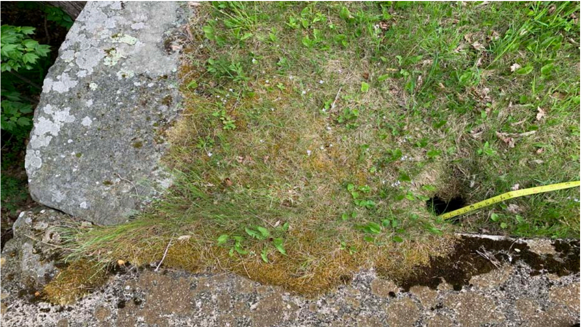
Photo 8: Void in right crest adjacent to the right spillway training wall.
