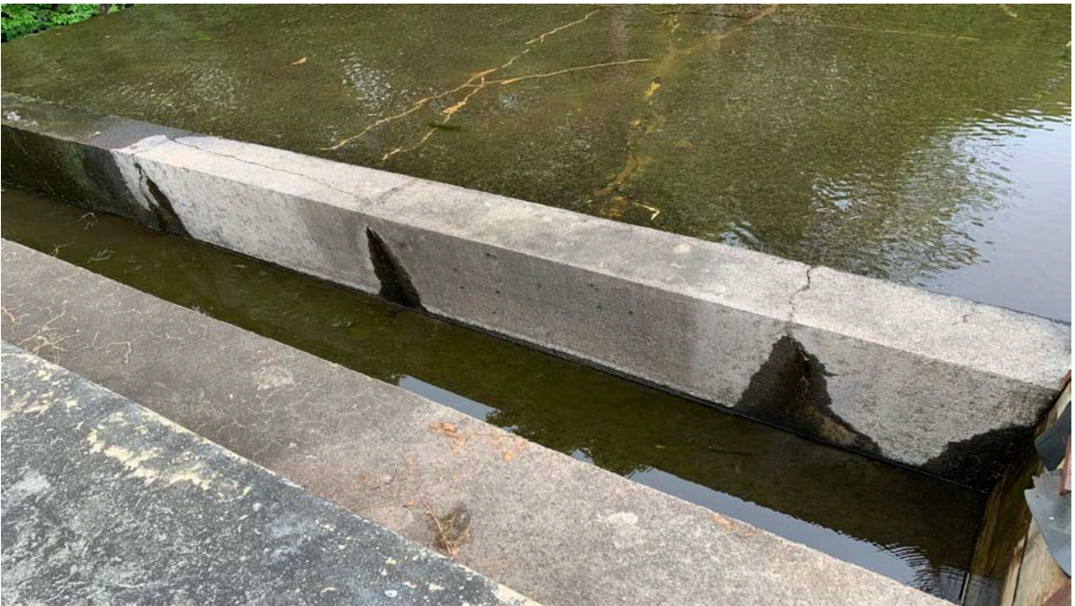
Photo 12: Shared wall between primary spillway and low flow sluiceway. Multiple cracks were observed with seepage through the cracks.
