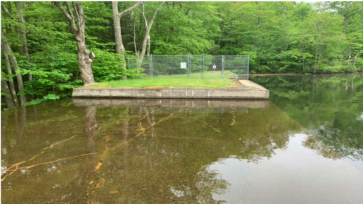
Photo 14: Primary spillway from the left crest – Cracks shown in spillway had been repaired from previous grout repairs. No deficiencies to note during this inspection.
