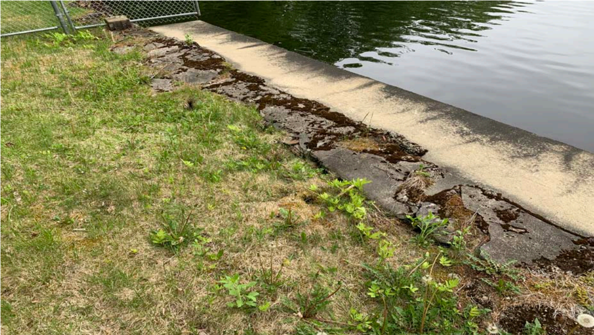
Photo 5: Upstream face between the spillway and the fence on the right crest – Multiple small voids/animal burrows were observed in this area.
