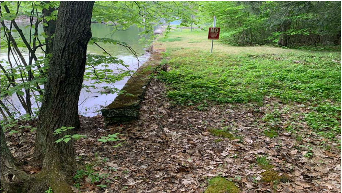
Photo 4: Right upstream face of the dam looking toward the spillway – The upstream wall was leaning outward.
