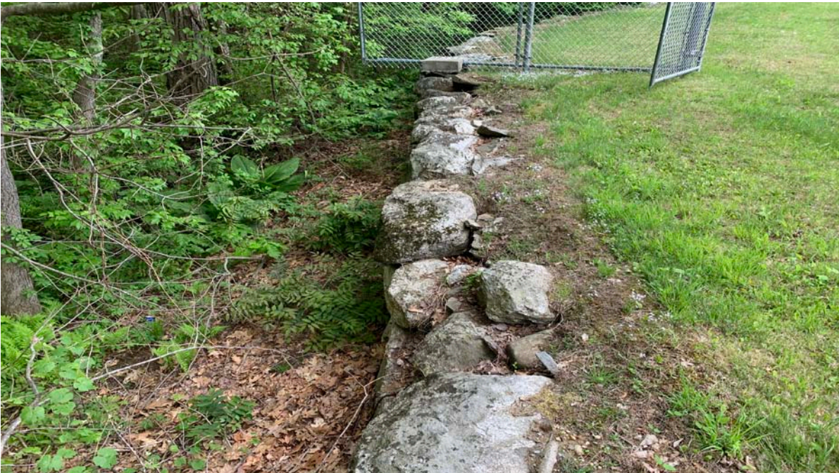
Photo 10: Left downstream face from the left abutment – Missing cap stones along the top of the wall in multiple locations. Heavy vegetation was observed within 20 feet of the toe.
