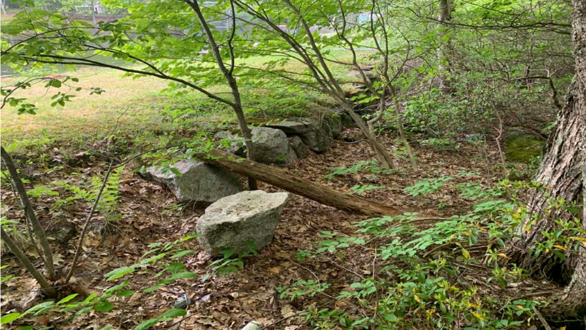
Photo 9: Right downstream face from the right abutment – Missing cap stones along the top of the wall in multiple locations. Heavy vegetation was observed within 20 feet of the toe.
