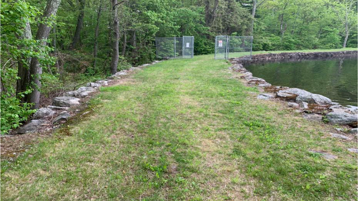
Photo 7: Left crest from the left abutment – There was some thin vegetation along the crest as well as some shallow tire rutting. Note the gate located across the crest.
