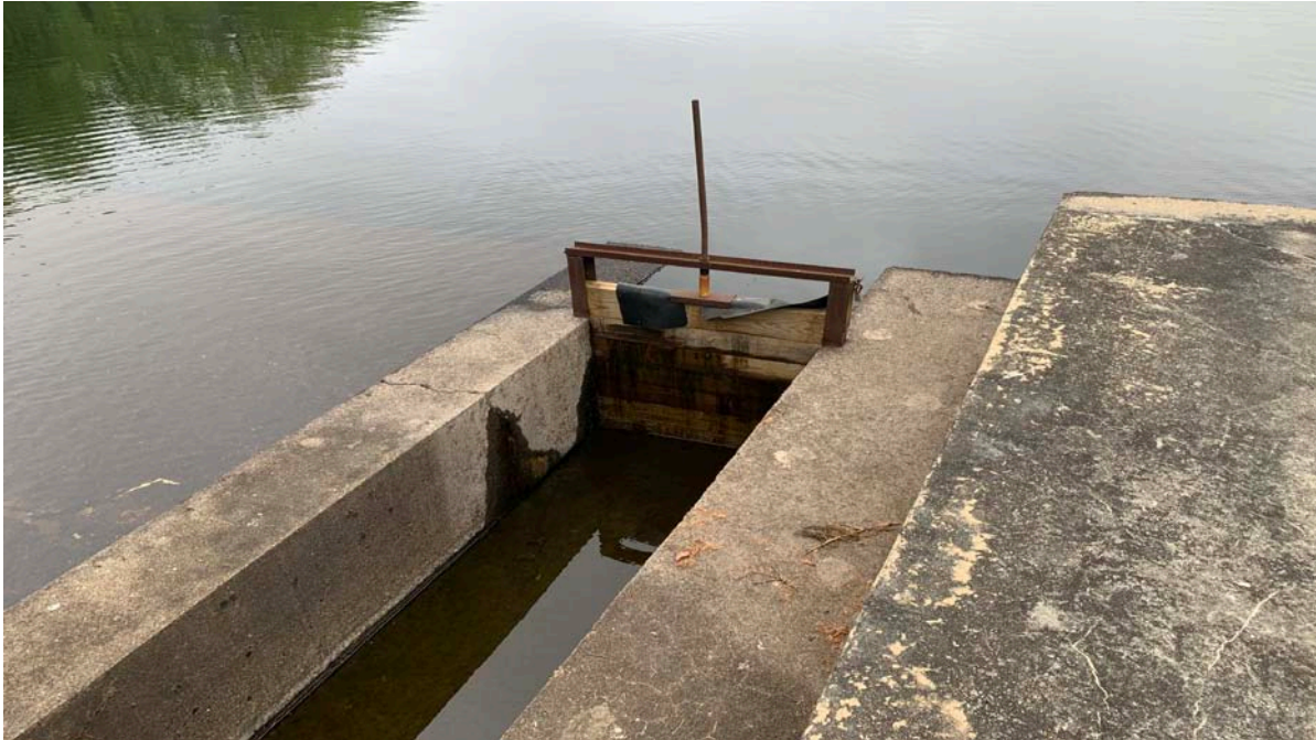
Photo 13: Inlet to the low flow sluiceway – Weir boards were in place at the time of inspection. Weir boards were recently replaced.
