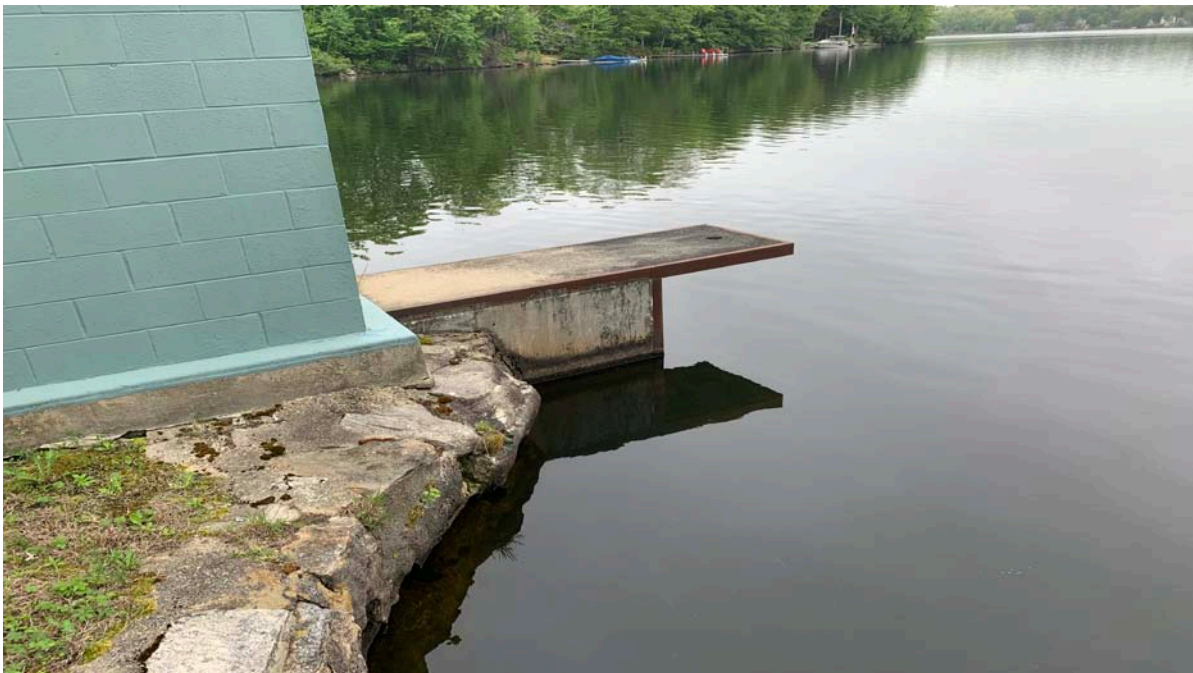
Photo 16: Access to the gate valve for the low level outlet is gained from this cantilevered platform that hangs over the upstream face of the dam.
